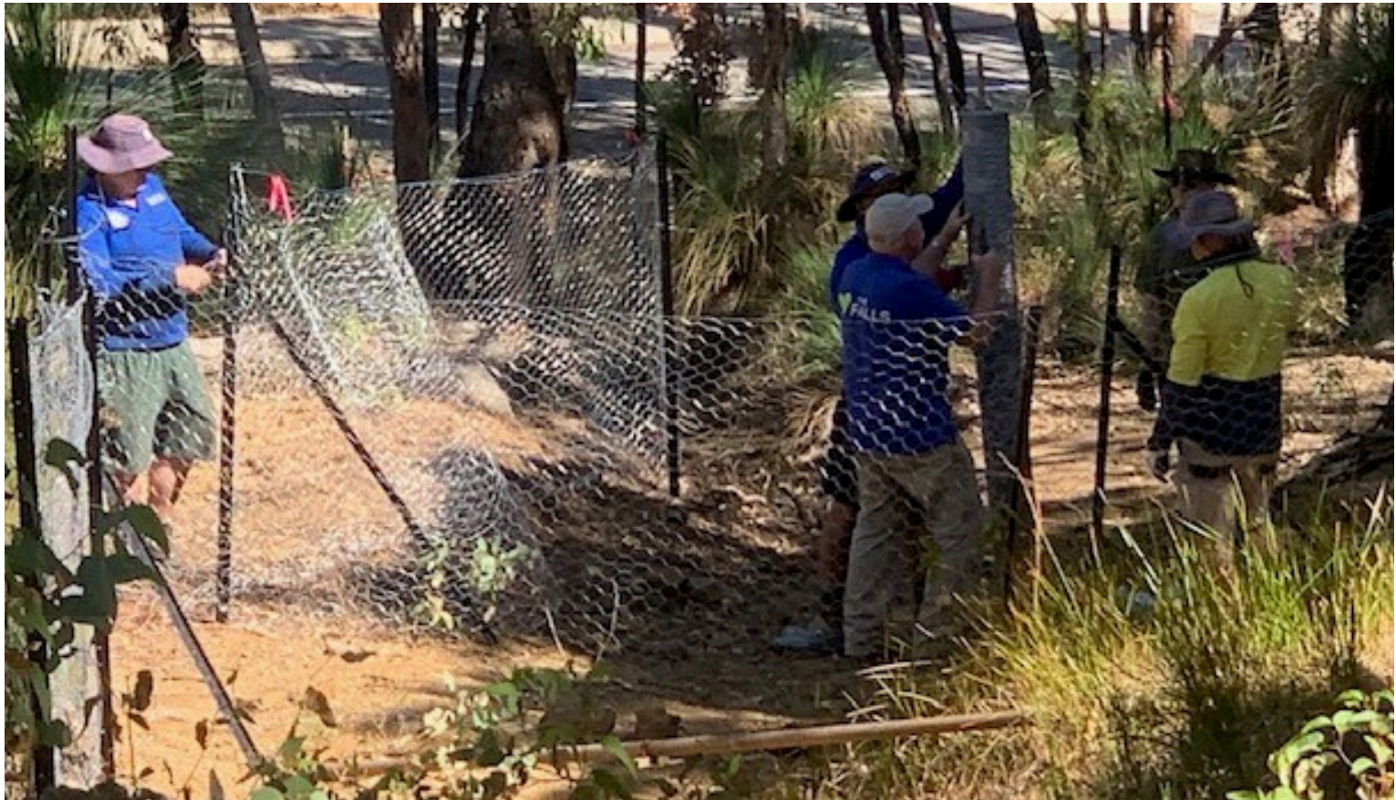
The fencing team hard at it in the erosion gully.
