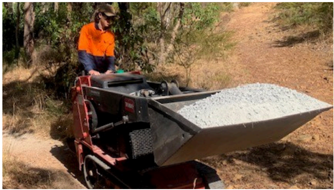
Hayden spreading road base for pathway upgrades.
