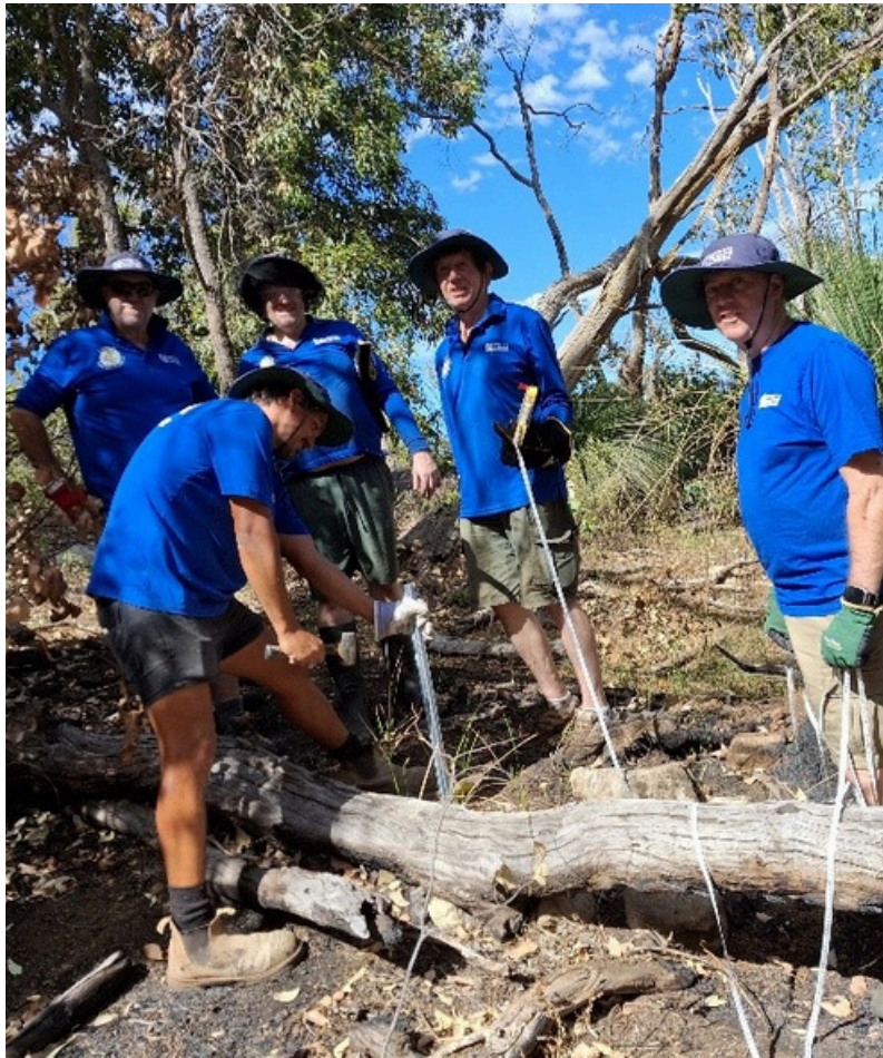
Clearing the path for new fencing.
