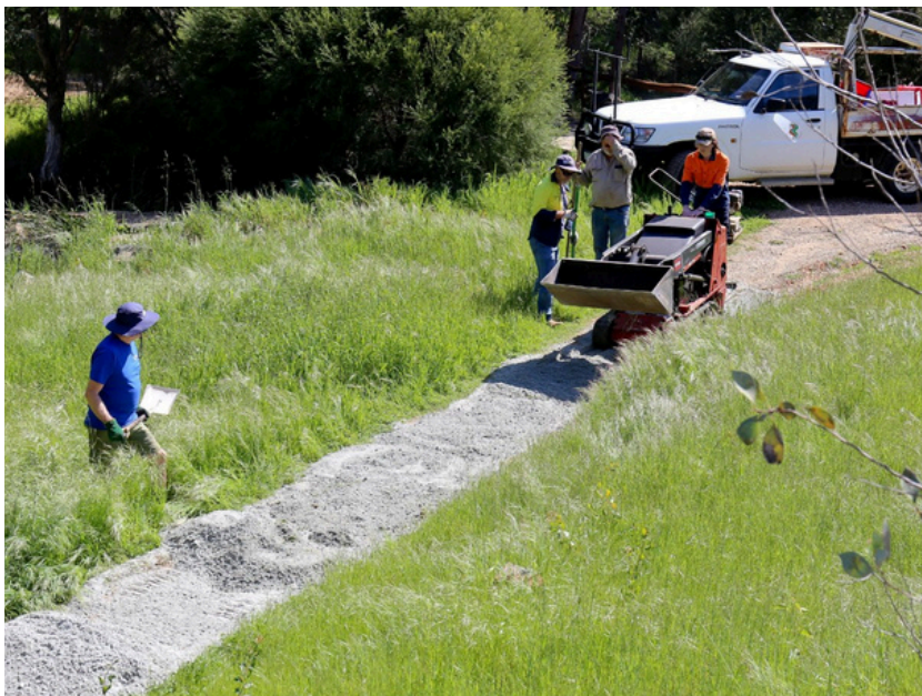
Erosion repairs on our pathway are a major project.
