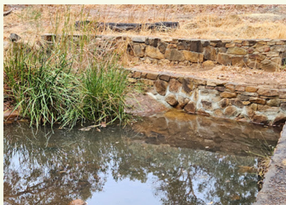
Dam wall stabilised
