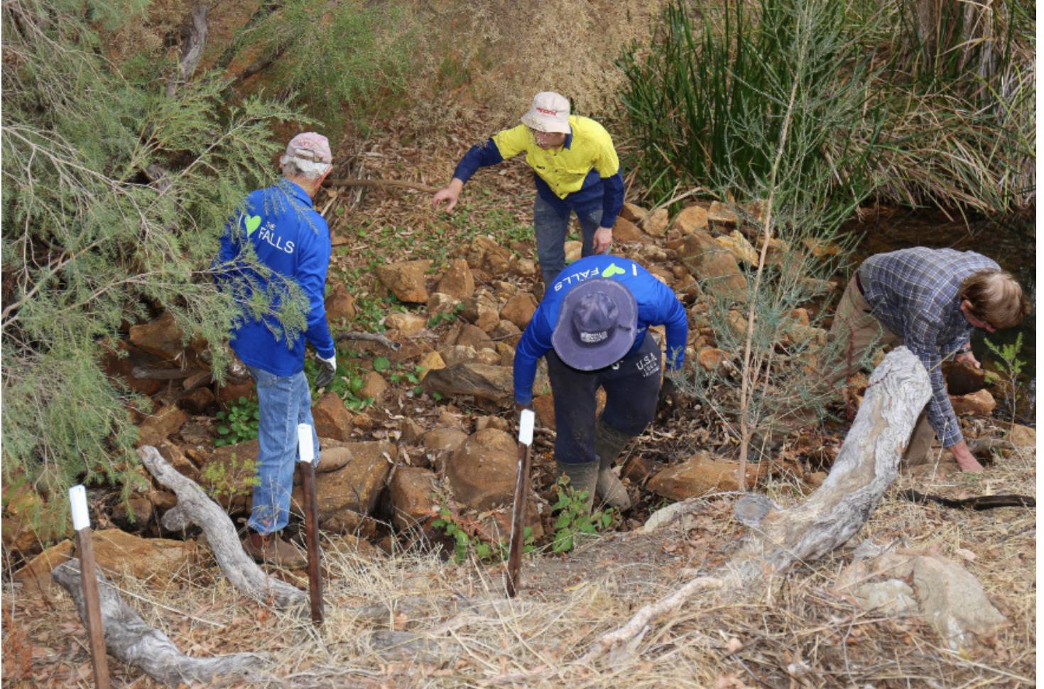
A team used rocks from the creek bed to protect the creek banks and improve flow.
