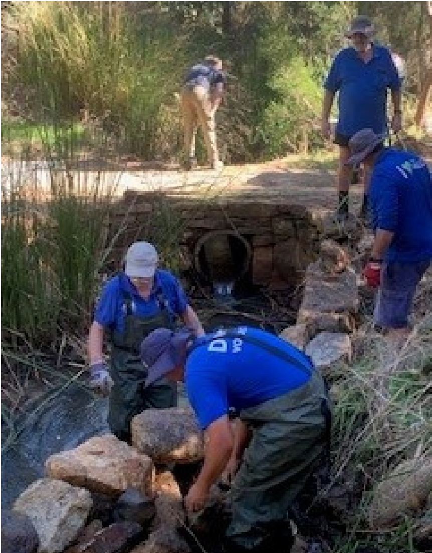
Some great masonry work by Jared.
