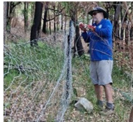
Paul putting the finishing touches to a cocky gate.
